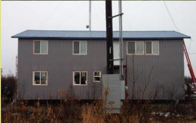
*The team was also able to put on a new and much needed roof. In the flying snow and icy conditions, it was a risky job. The men donned harnesses and tethered themselves to the roof and tackled the meticulous objective of removing the old roof and putting on the new. For days on end they worked in a stooped position on a slippery roof.*
